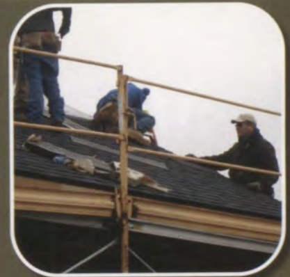
Mr. Handwerk watching as shingles are being put on the house
